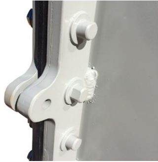
316 Stainless Steel Nut Inserts Installed
